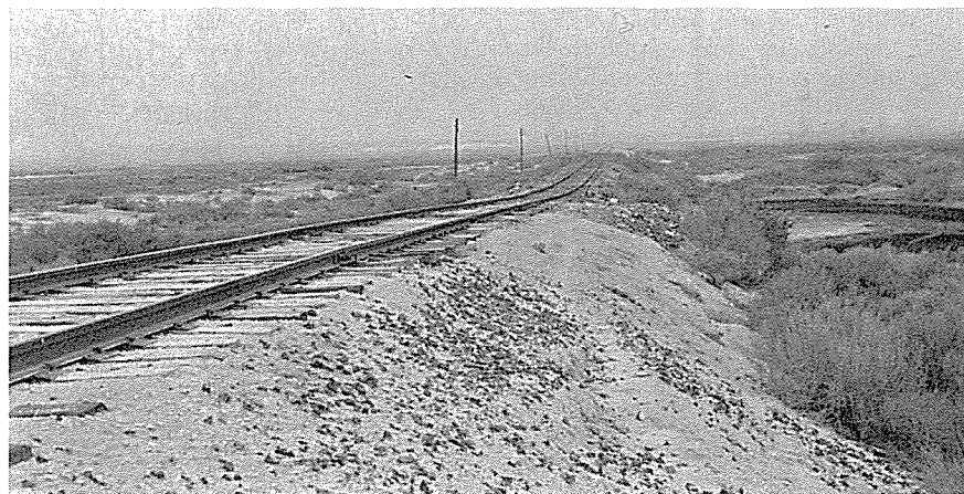
Subsidence along Sunset Railroad bed at waste water sump.
