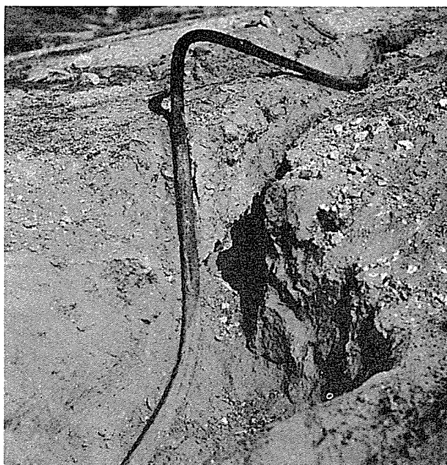
Abandoned 2-inch fuel line in north half of section 1, T. 32 S., R. 24 E., showing character of buckling it suffered at trace of Buena Vista fault. (From Thomas W. Koch, 1933)
