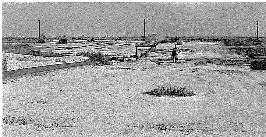
Subsidence at waste water injection well No. 8 in Section 5, T. 11 N., R. 23 W. Man is standing on capped well head.
