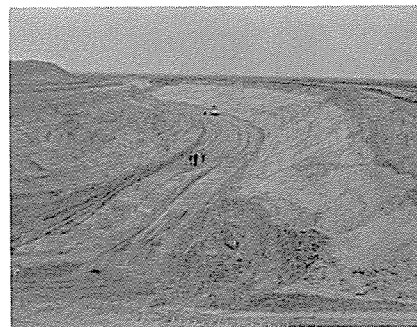
Survey crew in bottom of California Aqueduct canal prior to cement lining operations.
