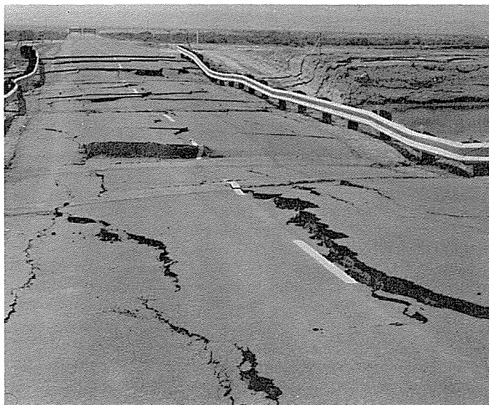
Cadet Road. Road damage due to compaction of soils causing subsidence.
